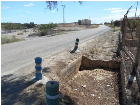
OBRA DE DRENAJE TRANSVERSAL: 2 TUB. ARCO Ø500mm
